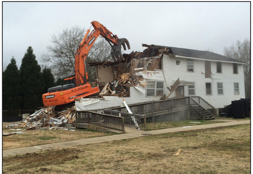
Soldiers Plaza, Bldg. 2602, a World War II wood building used most recently as an administrative facility, is demolished at Fort Benning, Georgia, under the Facilities Reduction Program.
